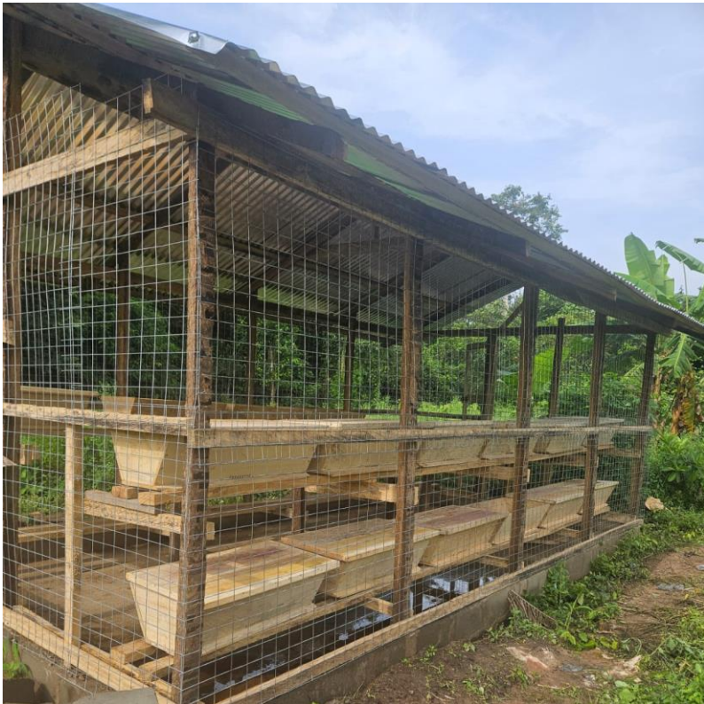
Figure 4. Hodzo-Achianse bee house and scientific bee boxes constructed to consolidate hives in MLS group-owned orange groves, and to protect beehives from fires due to slash and burn agriculture (Courtesy of Dickson Asase, 14 October 2025).
